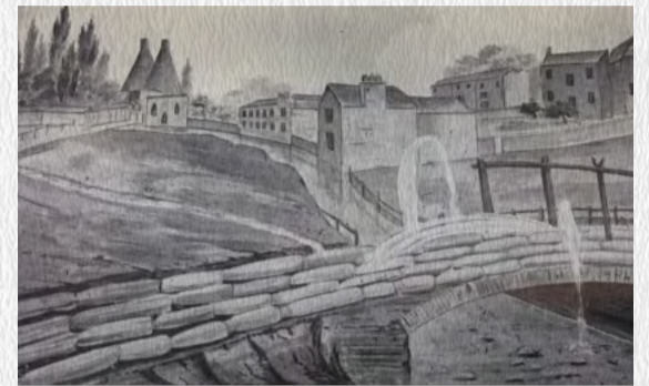
The conduit passing over the River Fleet
